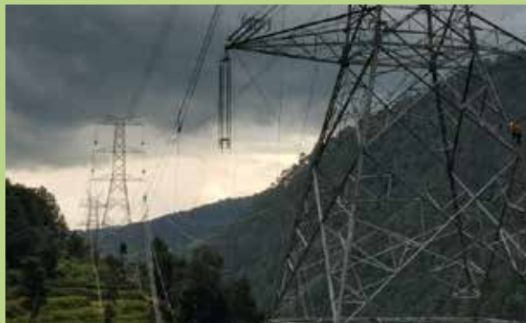
› High Voltage (400 kV) Transmission Line in High Altitude (2,716 m), Tamakoshi (Khimti) – Kathmandu TL Project.
