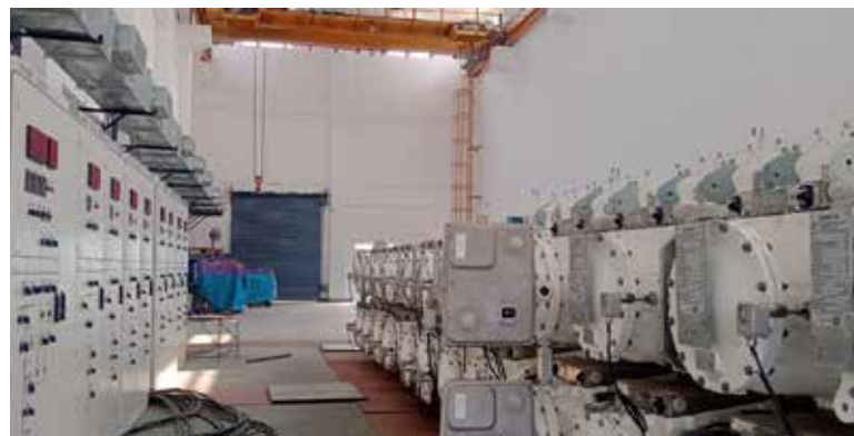
132 kV AIS to GIS conversion, GIS module erected at Gohpur site → Gantry structure erection & Transformer installation under progress at substation under AEGCL project Switchyard → Equipment erection works under progress for AEGCL project ↓
